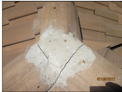
(3) Cracked/damaged mortar pack(s) noted - Review
