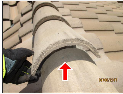
(3) Cracked/damaged mortar pack(s) noted - Review
